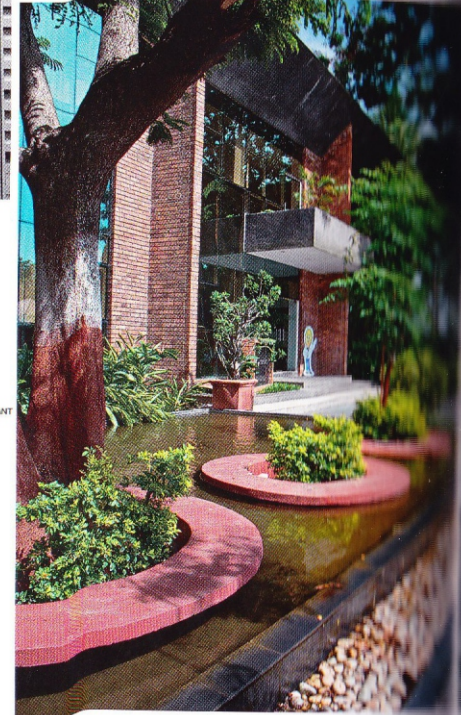
Photographs showing the pre-cast ferrocrete planter supports made on site
