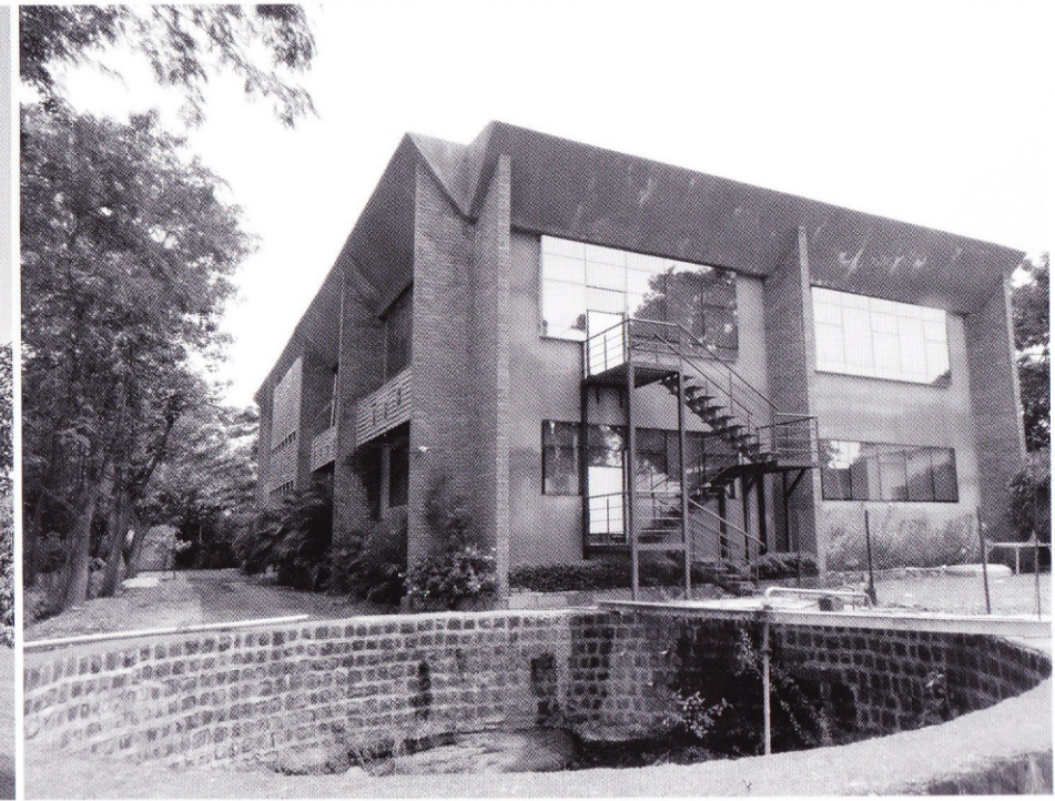
Existing well is retained and used for rain water harvesting and the treated water is used for drinking purposes.
