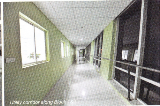
Utility corridor along Block 1&2
