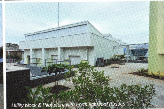
Utility block & Pilot plant with north light roof trusses
